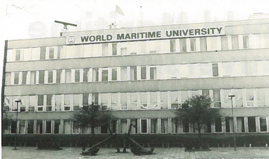
A general view of the World Maritime University building, which was donated by the City of Malmö.
