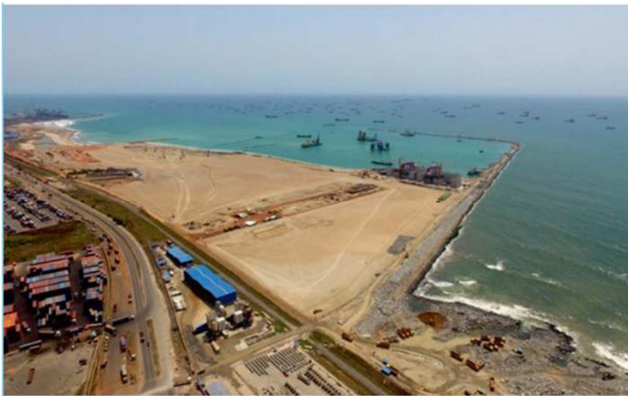
Figure 2.3 1: Overview of Tema container terminal
