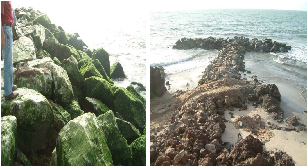
Figure 15: Revetments & T-groynes on the beachfront of Cape Point
