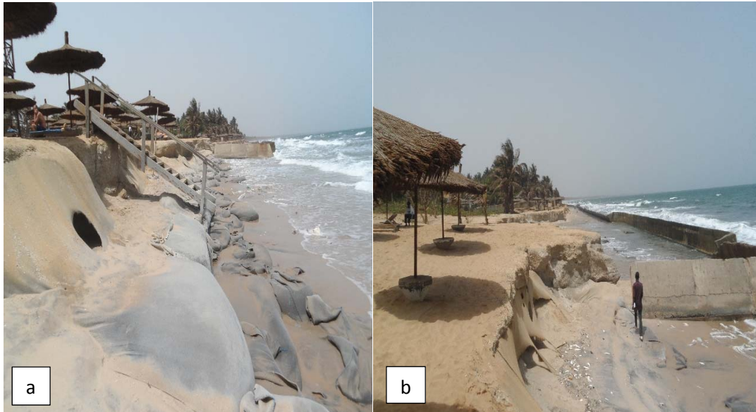
Figure 9: Unsustainable adaptive measures for erosion control
