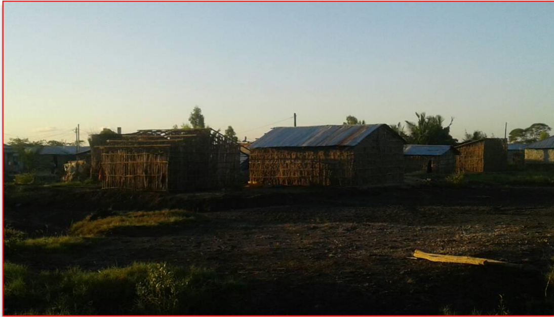
Figure 8. Houses on Mangrove Land at Chuabo- Dembe
