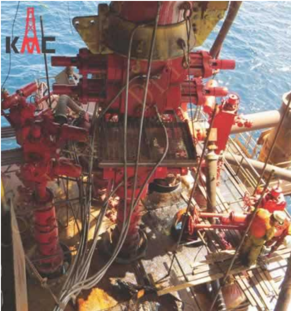
Figure 5: Image of Ocean Drill BOP being deployed
