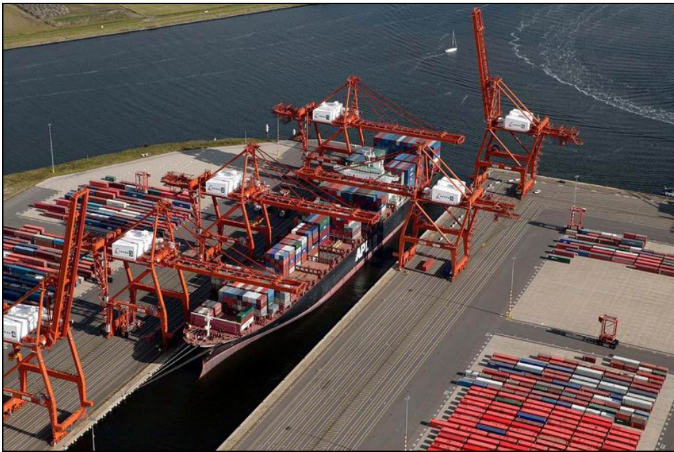
Figure 57 : Water basin in operation
