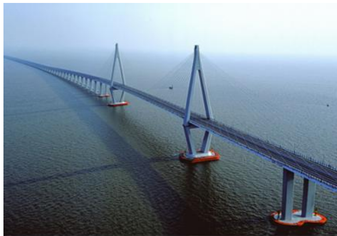
Figure2.4 North main navigable span of Hangzhou Bay Bridge
