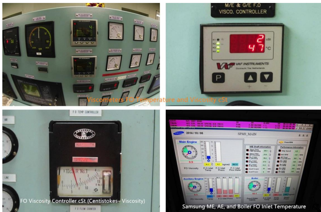
Figure 3.3 - Several common fuel temperature, viscosity meter
