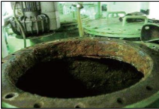
Figure 10: rust status of the aeration tank
