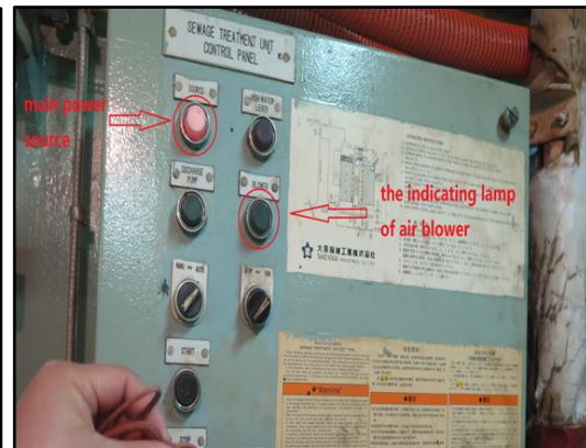
Figure 16: the control panel of treatment plant.
