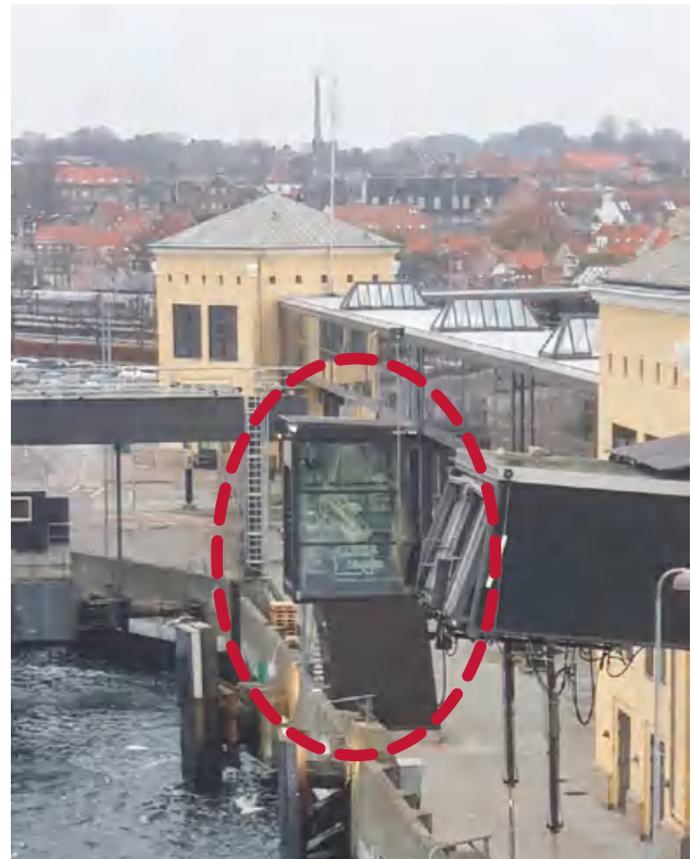
FIGURE 5.3.12 Fully-automated, laser-controlled robotic arm for charging batteries in Helsingborg, Sweden.
