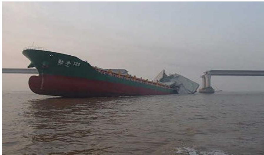
Figure.4 - “Qinfeng 128” Impacted the Jintang Bridge
