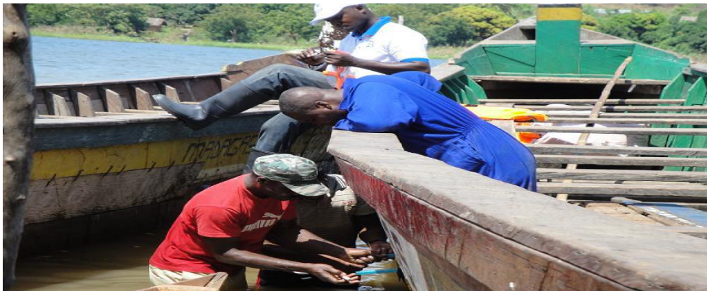
Figure 11: GMA surveyors marking boats with loadlines (Source: Ghana Maritime Authority, 2010)
