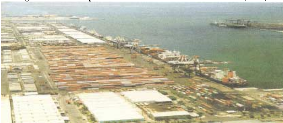
Figure 1.2 Helicopter View of the North and South Terminals (KTO)
